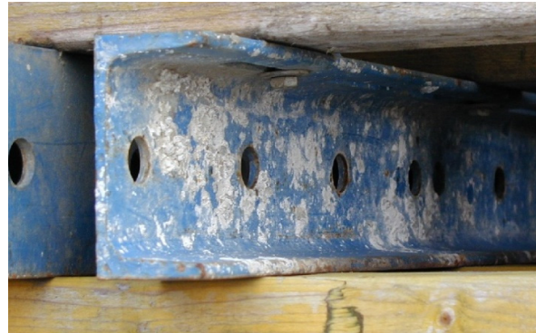
Photo 7 Permissible concrete debris on steel waling
