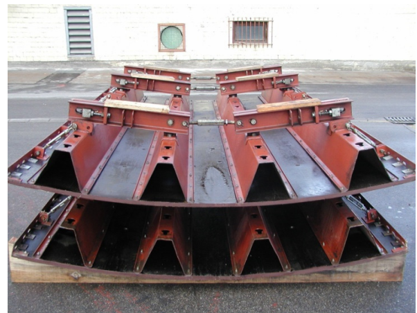
Photo 9 Use of timbers for stacking formwork panels
