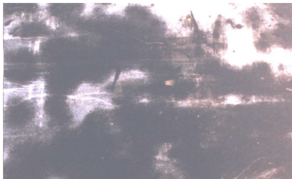
Photo 17 Permissible cleaning condition formlining
